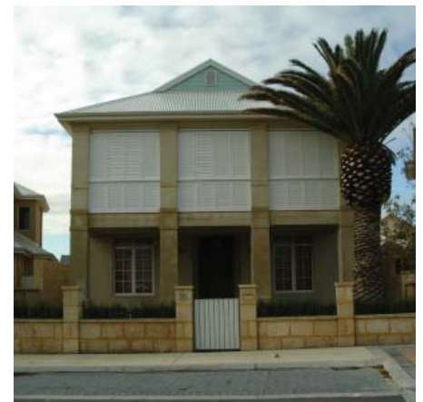
Operable sunscreens protecting west face
