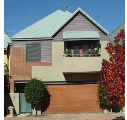
Balcony and windows overlooking rear laneway
