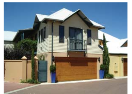
Openings providing outlook over laneway.
