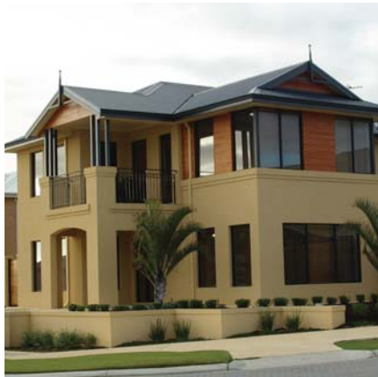
Articulated secondary street elevation.
